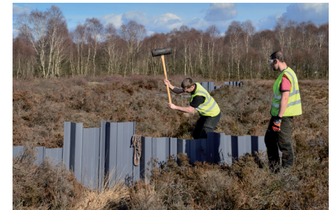
Blocking old drainage ditches to raise water levels on lowland raised bog, Flanders Moss, central Scotland.
