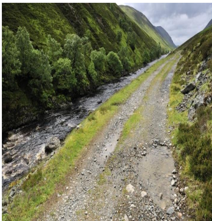
Existing upland track. Note that a level of maintenance will be required to prevent ponding and erosion / run-off.
