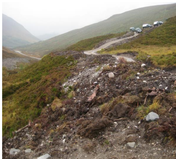
Potential erosion and run-off from neglected track edges
