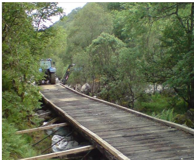
Temporary floating boards construction avoiding sensitive habitat beneath.
