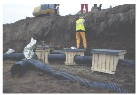
Above: plan of a medium size Type 1 Design artificial sett. *Right*: Type 1 Design artificial sett under construction, A97, Aberchirder, Scotland (Grampian Badger Surveys for Aberdeenshire Council 2000).
